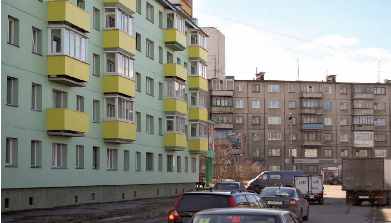
“Krutsovky” blocks in Murmansk. Note the new facades (light green) with extra insulation. Photo: Odd Iglebaek
