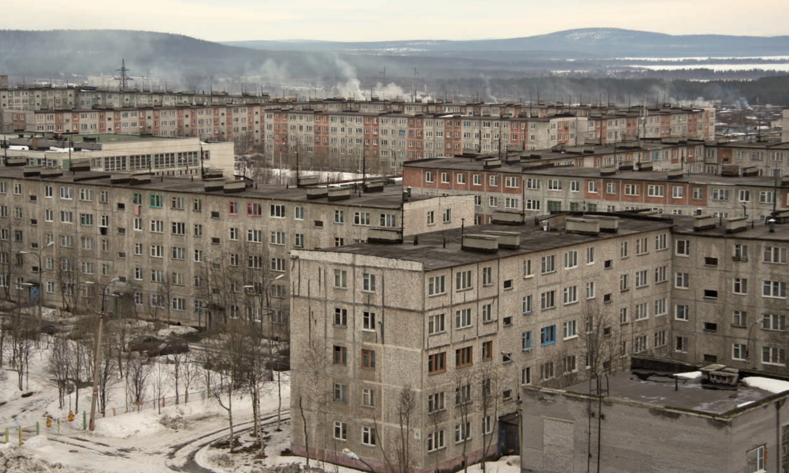
Typical Krutsjovky -style housing in Northwest Russia, here from Apatity. Note the different standards of windows. Photo: Odd Iglebaek
