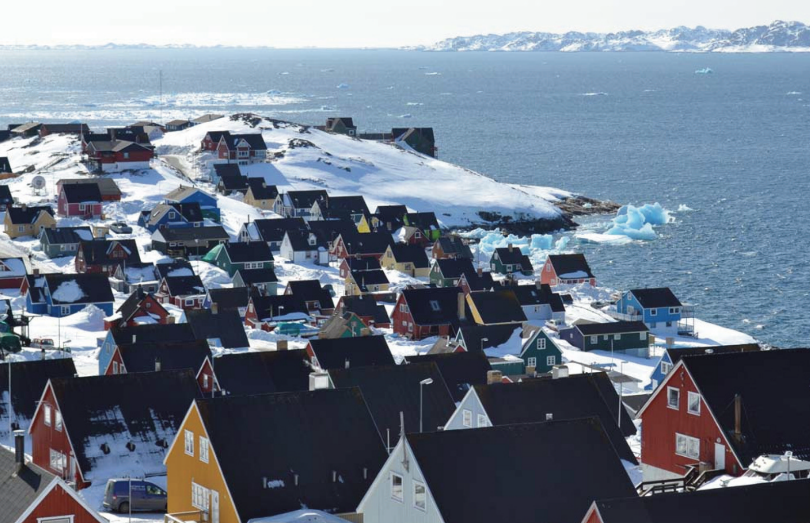
Myggedalen in Nuuk provides a typical example of the rapid growth of the private housing market in the Arctic. Photo: Minna Riska
