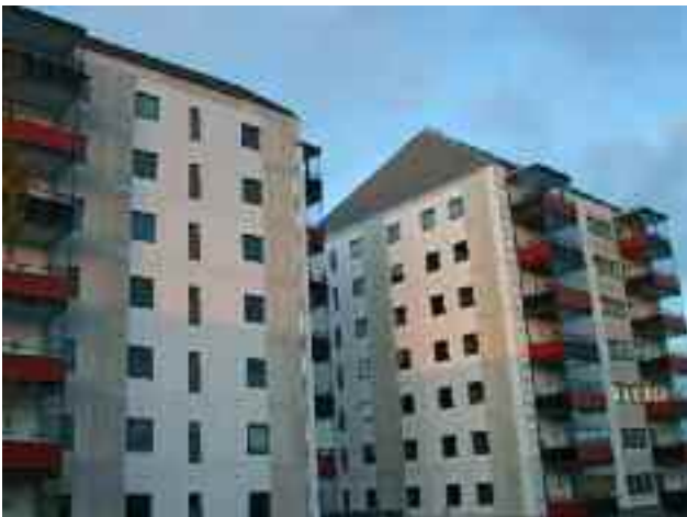
Part of the "greening" process in Växjö is the drive to build passive houses and large wooden structures. Top to left shows the record eight storey high wooden houses in Limnologen. Bottom left is Portvakten Söder built in 2008 combining high-rise wooden structures with the passive-standard. Outside cladding is cement-fibre plates. Inside is gypsum. Window-photo to show thickness of finished wall. Top right Erik Hallonsten, Senior Manager of Hyresbostäder Växjö shows model illustrating the insulation-construction in the passive house. All photos: Odd Iglebaek
