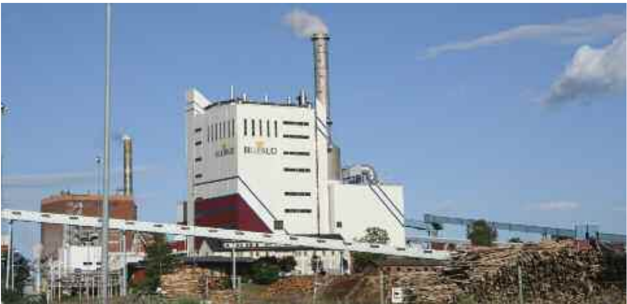
Gruvöns Bruk/ Billerud in Grums, Värmland. Photo: Odd Iglebaek
