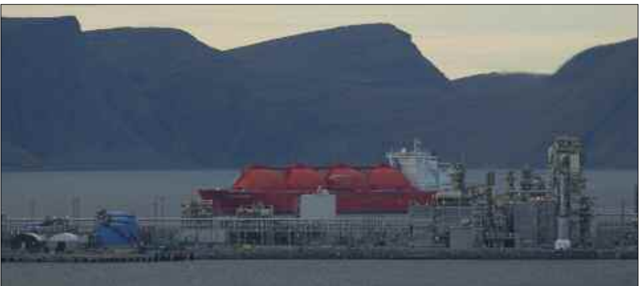
Part of the huge gas-processing installations at Melkøya with LNG-tanker. Photo: StatoilHydro
