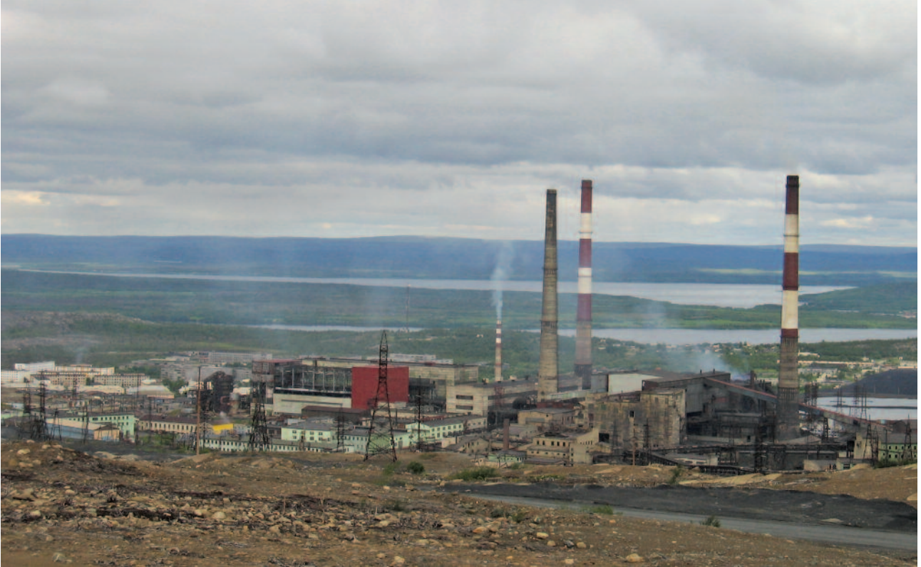
Northern peripheries, here from Nickel in North-West Russia. Photo: Magne Kveseth
