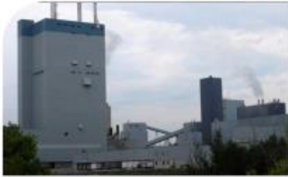
First commercial installation of Lignoboost™ lignin recovery, Domtar
