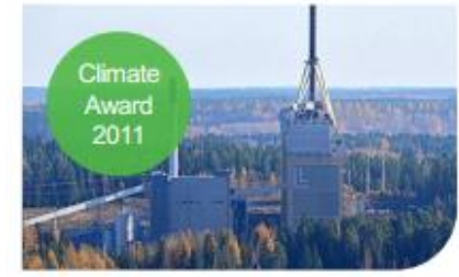
World's largest Waste-to-Energy Gasification Plant, Lahti Energia
